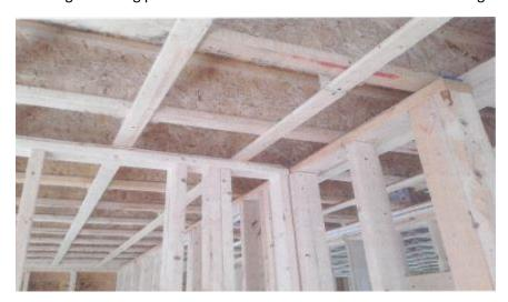
All fixtures such as light cans and exhaust fans are attached to the furring, not the joists.
